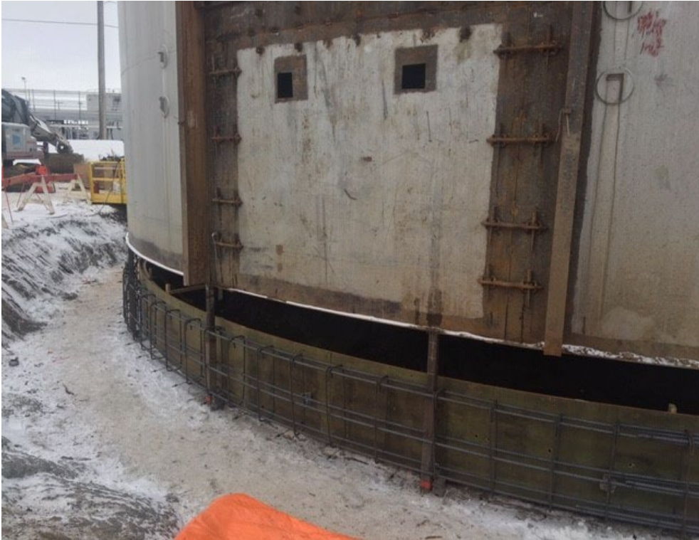
New concrete ringwall foundation under existing tank
